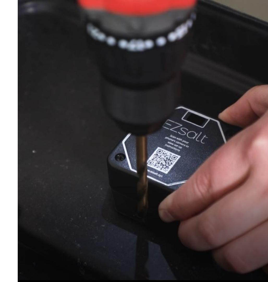
Using a 1/4in drill bit, line up the tabs on the EZsalt
